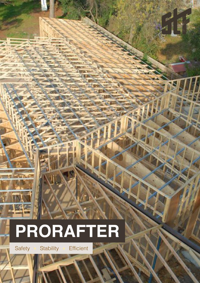
**ProRafters** are a new engineered wood product that combines highly reliable plywood and LVL to form a composite 'C' section beam. The composite beam allows an economical formation of a wide variety of geometric shapes, ranging from linear tapered, top edge curved and to fully curved. refer to page 2 for other geometries.
